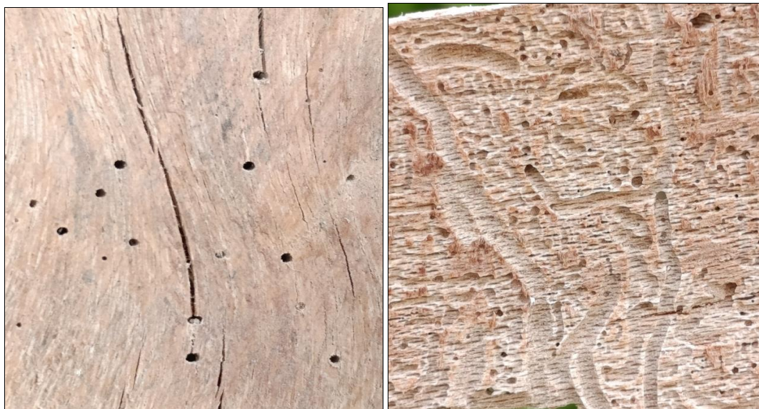
Fig 3: Damage caused by beetles
