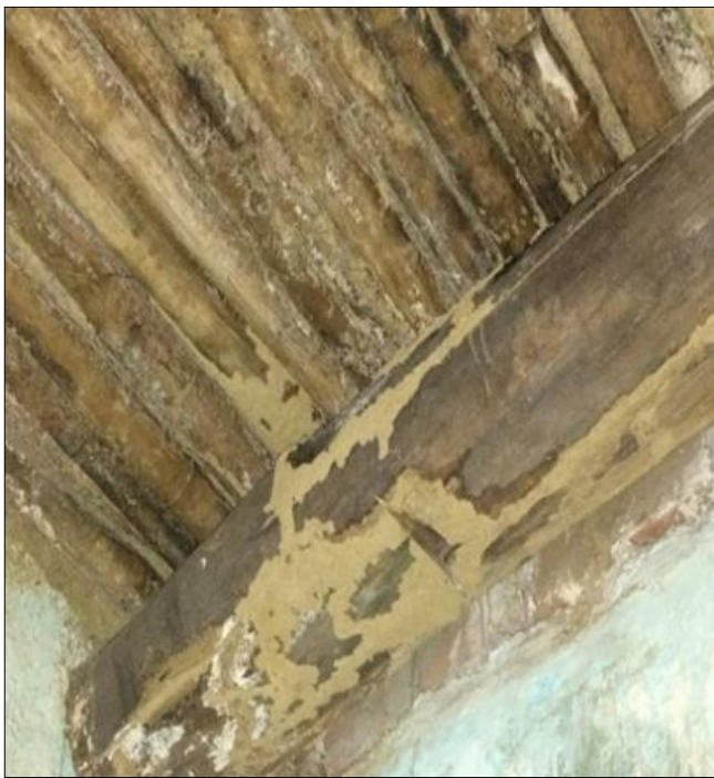
Fig 2: Termites attack on wood
